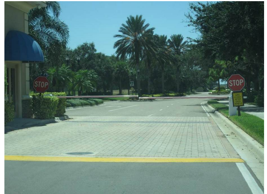
Both Stop Signs too short at exit at Guard House on Stone Harbour Loop
